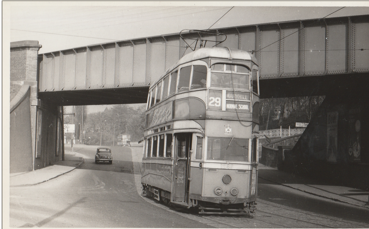
1245 on service 29 inbound from Broomhouse just going under the railway bridge at Mount Vernon.
